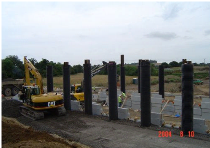
Reinforced Earth Abutments under Construction at Scotch Green Road Underbridge
