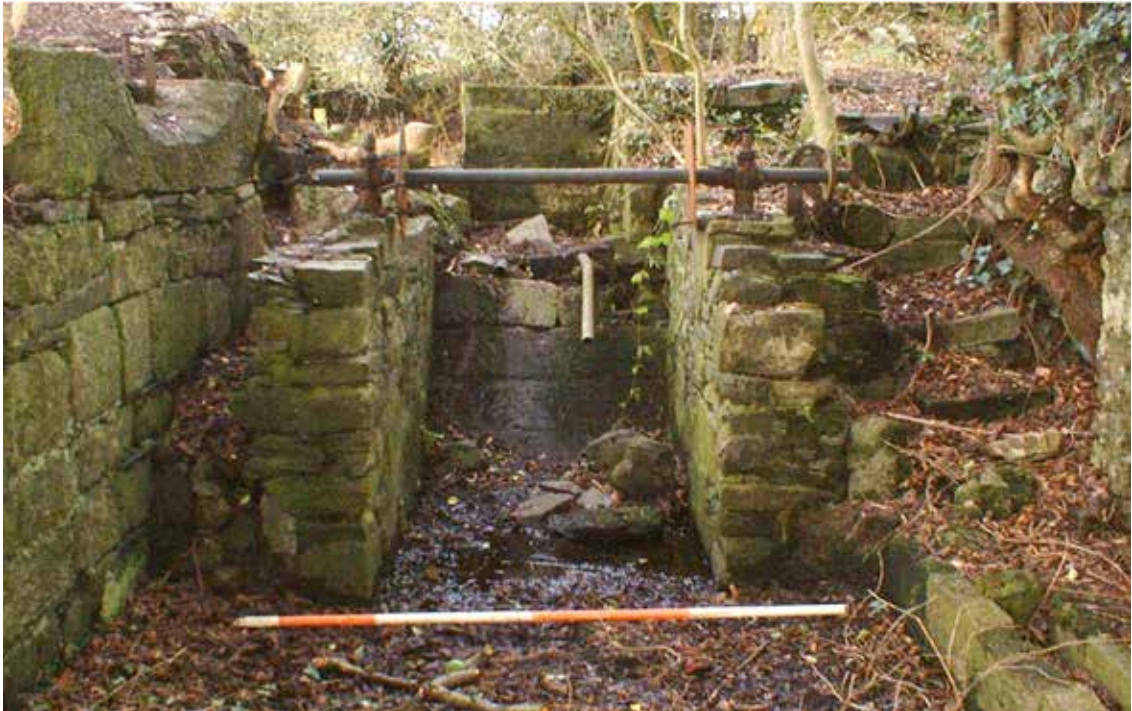
Illus. 7.5 Scotch Green Mill. North-facing view of the wheel-race. The water was delivered through the sluice over a stone-lined channel, and down a stone ramp to an undershot waterwheel (IAC Ltd).
