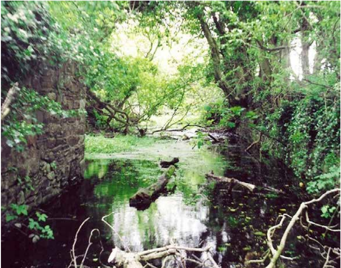
Illus. 7.2 Scotch Green Mill. Building remnant (left) and mill-race looking north-west towards the millpond (IAC Ltd).
