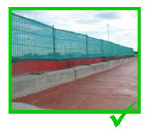
Side netting should be installed to prevent debris from falling onto areas of activity below, including water courses.
