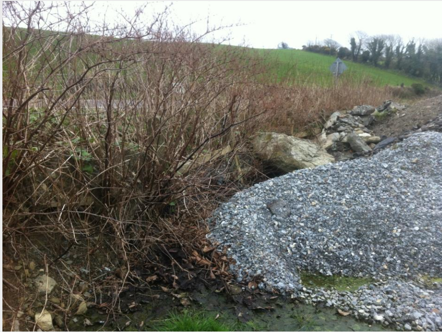
Japanese knotweed adjacent to road material (BAD)
