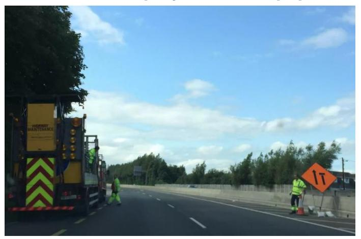
Operative not allowing sufficient time to cross live carriageway
