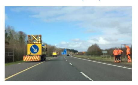
Advance warning signs installed from deployment vehicle protected by IPV
