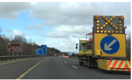
Lead in taper installed on live lane protected by IPV
