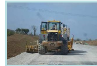
N22 Tralee Bypass: Laying of Cl. 804 with adapted machinery.
