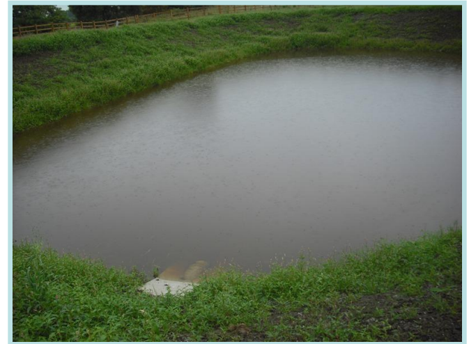
N21 Castleisland Bypass: Example of an attenuation pond.
