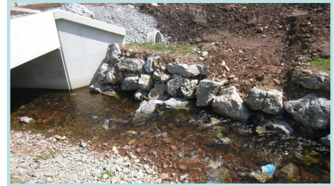
'Rock armour' training works.
