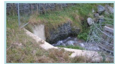
Reinforced concrete headwall with gabion training works.
