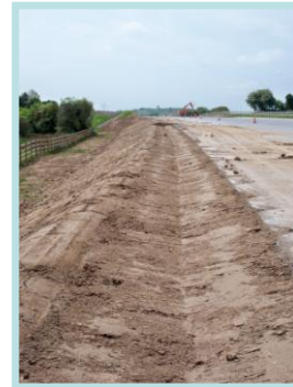
M17 Gort to Crusheen: Finished topsoil profile.
