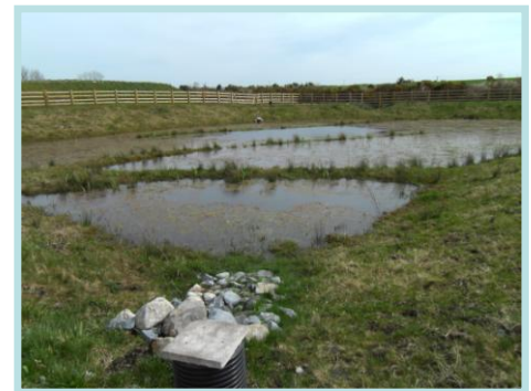
M18 Gort to Crusheen: Hybrid Wetland with sediment forebay.
