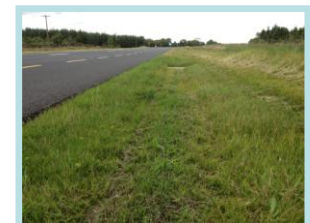
N52 Carrickbridge to Clonfad: Finished GSWC.
