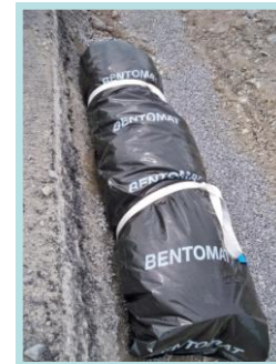
Use of Geosynthetic clay liners on M17 Gort to Crusheen.
