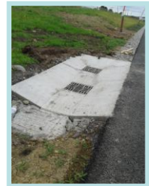
N5 Ballaghaderreen Bypass: Outlet.
