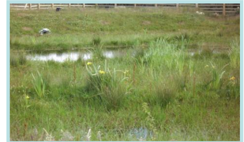
M18 Gort to Crusheen: Constructed wetland.
