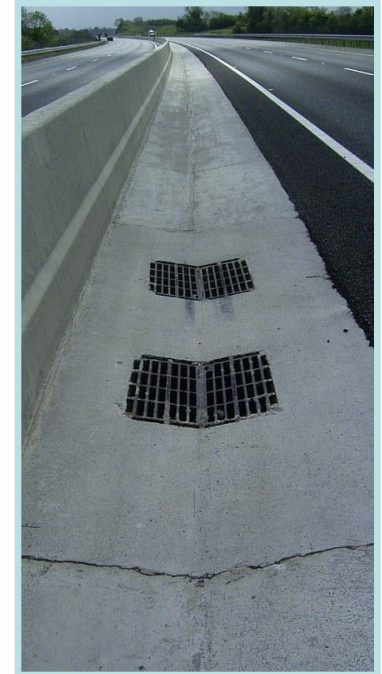
M3 Clonee to Kells: Concrete surface water channel and outlet.
