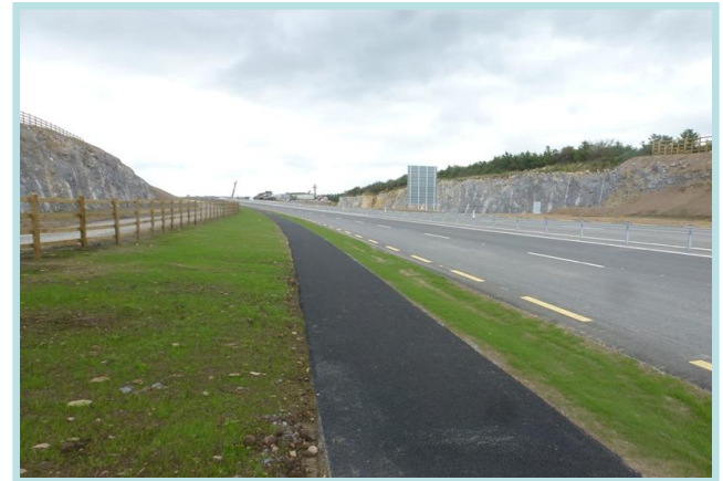
N22 Tralee Bypass: Grassed Surface Water Channel.
