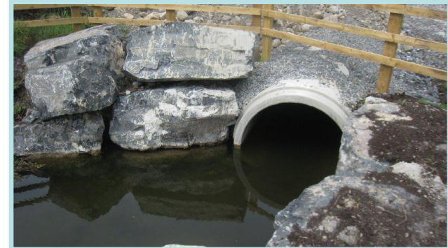
Example of 'rock armour' headwall.
