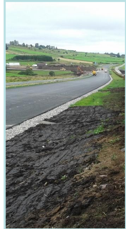
Combined filter drain on the N5 Ballaghderreen Bypass.
