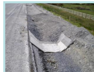
M17 Gort to Crusheen: Lined GSWC construction.
