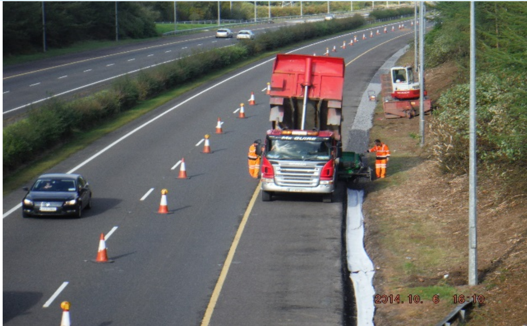
Filter Drain Remediation Works
