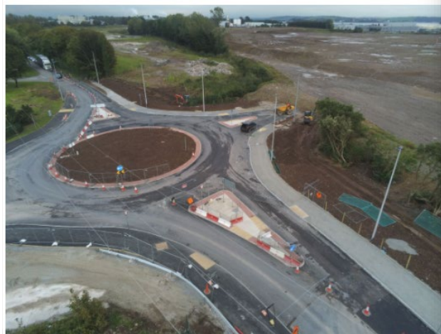
Aerial shot of the recently completed R623 roundabout
